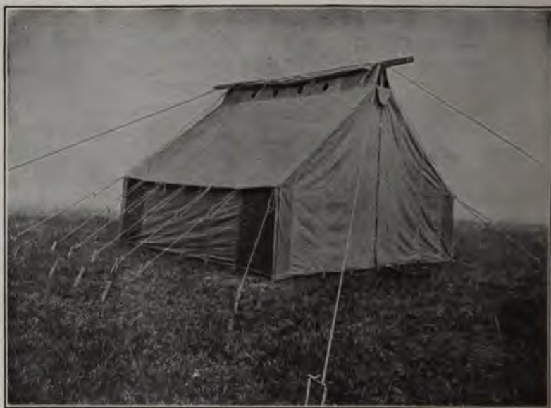
FIG. 194.—Hospital tent, tropical, showing ventilation of attic.
